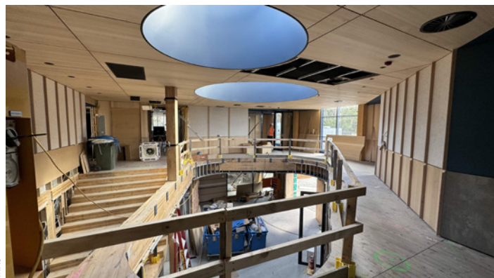
Images showing construction progress of the new teaching and research building at IMAS Taroona.
