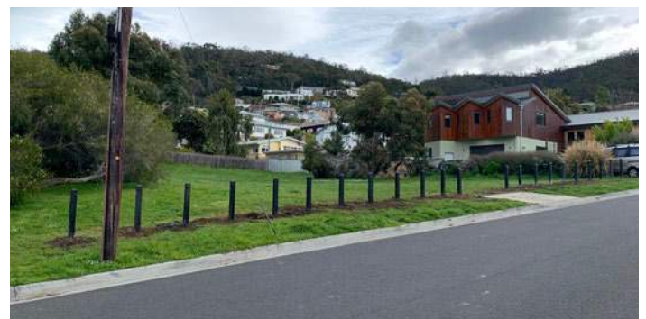
Recently installed bollards at Louise Hinsby Reserve
