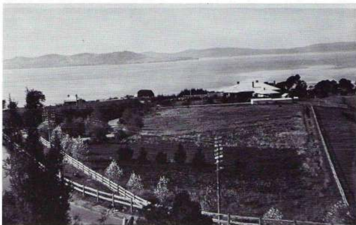
“Wartling”, now 12 Meath Avenue on the right and Retreat Farm, the home of Mr George Dixon, on the left.
