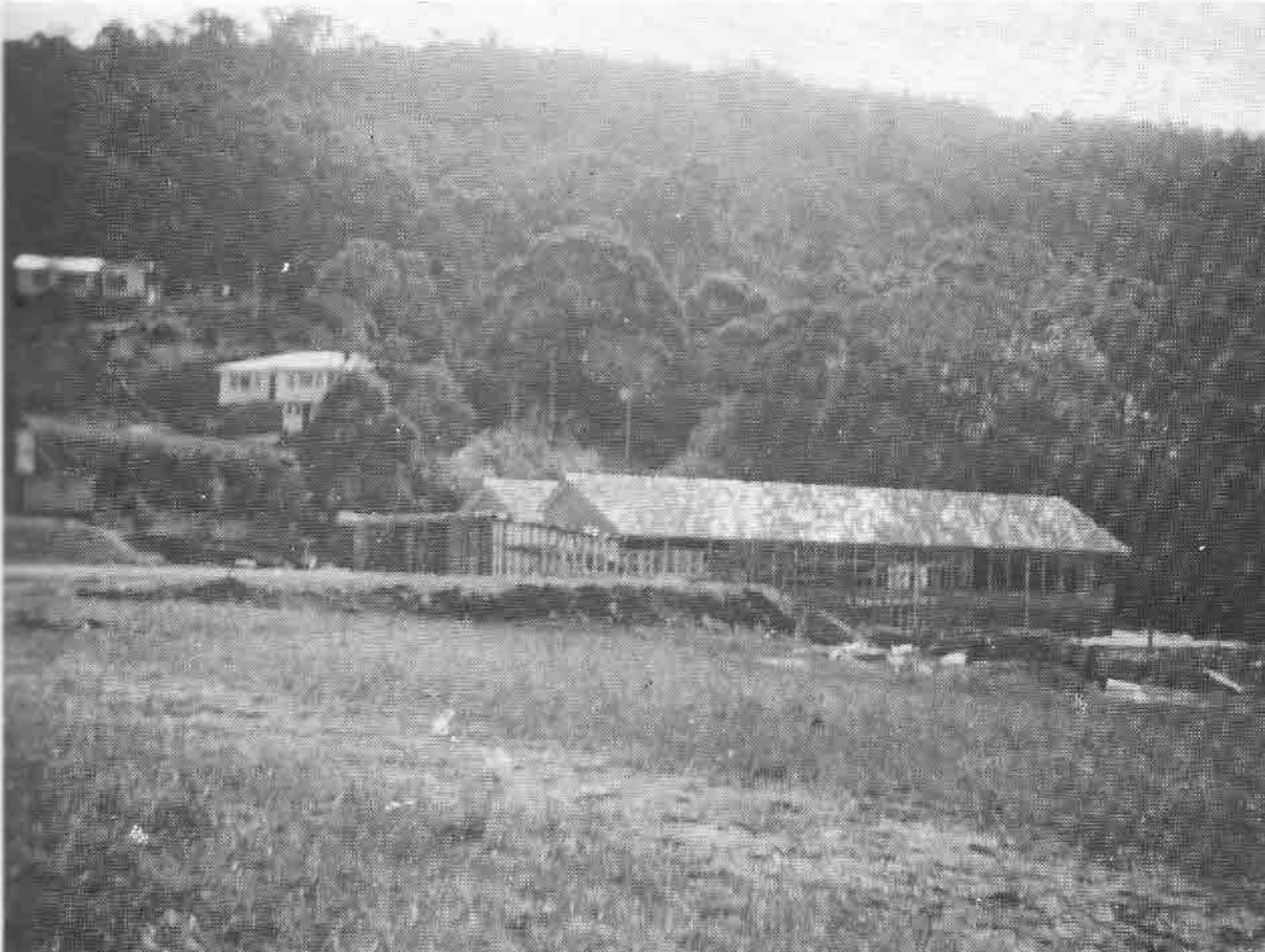
The new school under construction, 1960.
