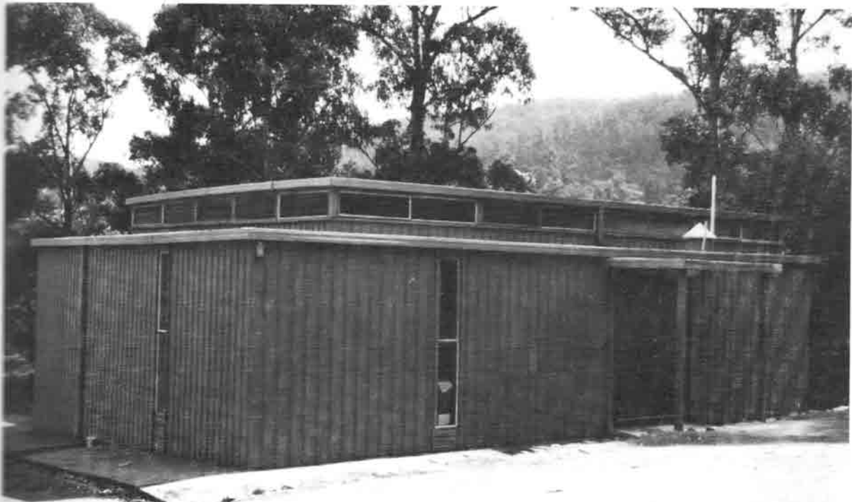
The Scout Hall taken in 1986, as rebuilt after the 1967 bushfires.
