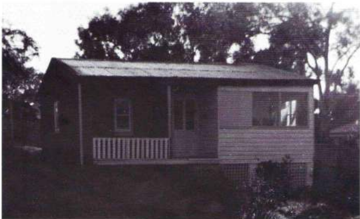
The Twelfth Apostle at Number 4 Seaview Avenue, Taroona, before demolition, May 1969.
