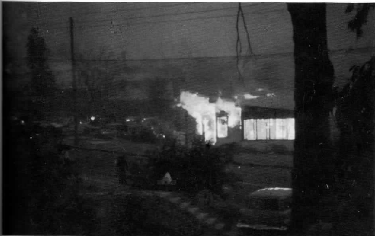
The Doctor's Surgery in Tarooma Crescent, burning down during the bushfire of the 7th February 1967. Note the Old Public Hall which stood on the corner of Tarooma Crescent and Channel Highway has already been consumed on the left.
