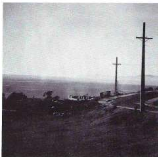
Illawong Crescent looking south, showing the foundations of number 16, the home of Drs Alan and Hilary Wallace.
