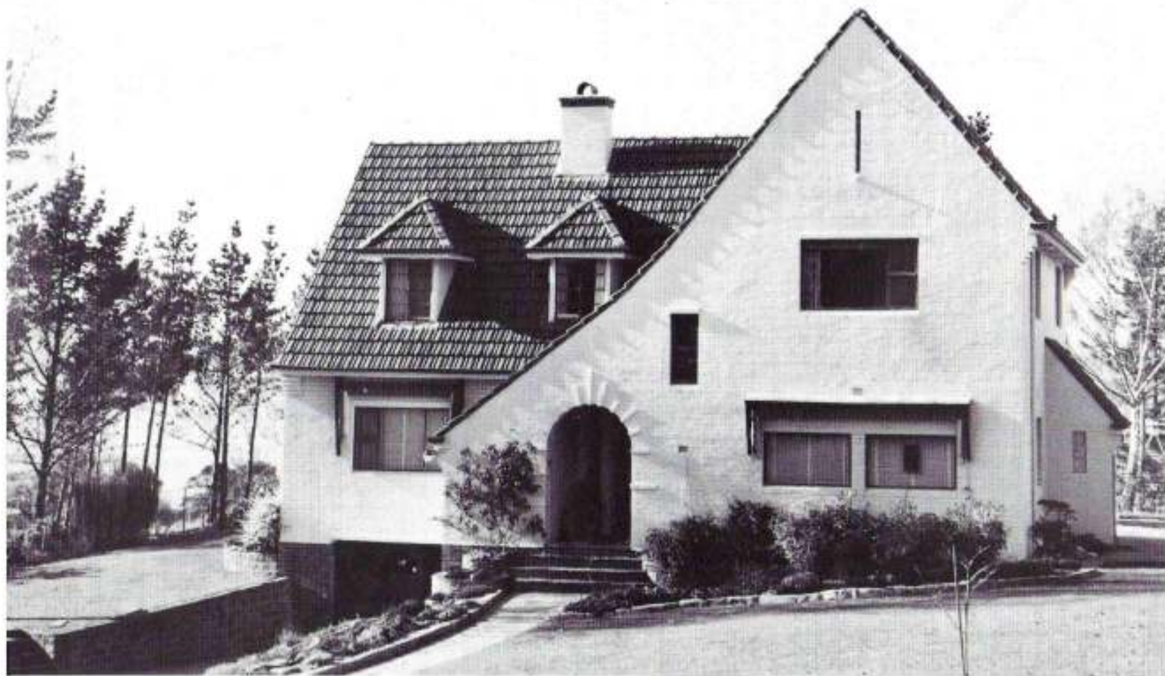
Number 26 Channel Highway, the home of Mr J.A.P.G. Boot.
