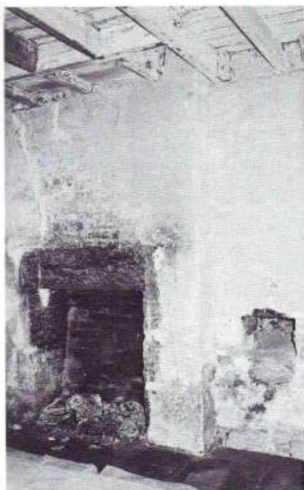
The ground floor kitchen at "Acton" before restoration, with the bread oven on the right, 1981.
