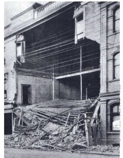
Collapse of the facade of Whitesides Building onto Liverpool Street in July 1923. The same building, a real warren with parts over 200 years old, is now known as the Bank Arcade.
