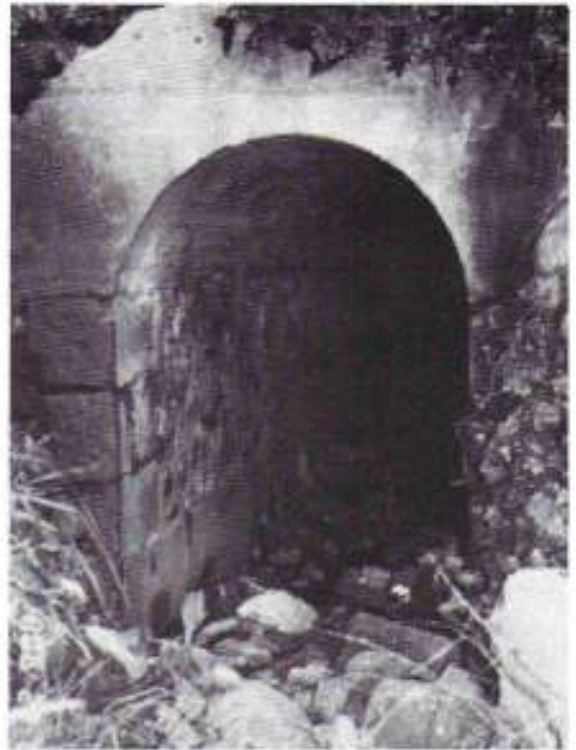
Entrance to the Churchill Road Tunnel.
