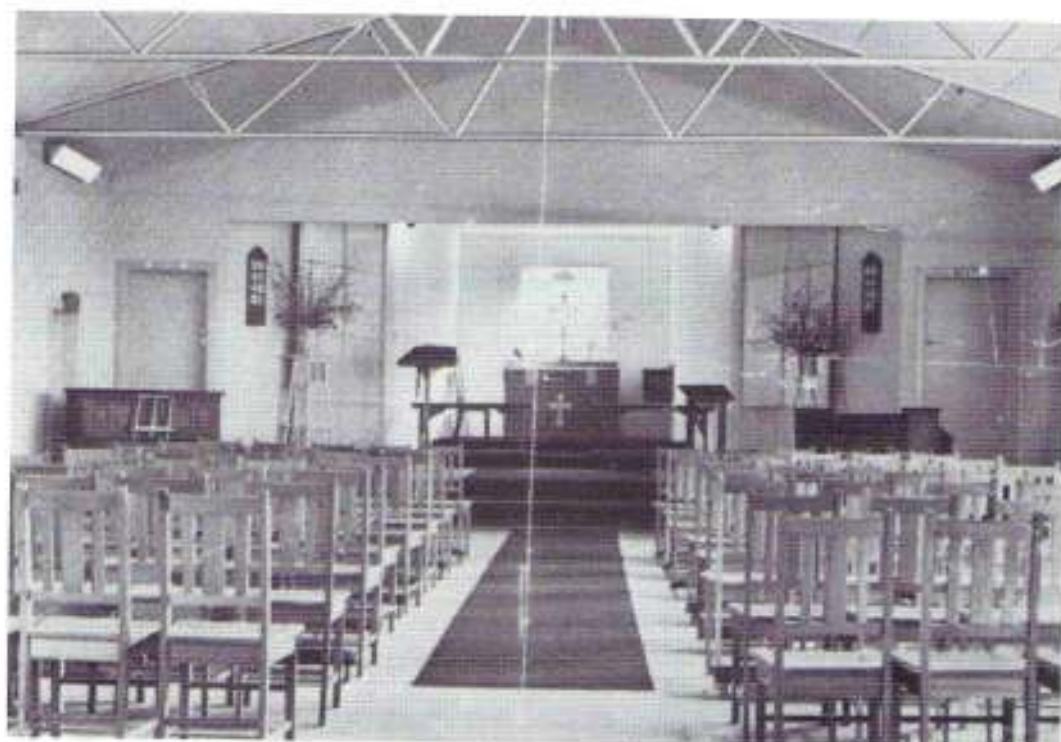
Stage and Sanctuary in the west end of St. Luke's Church Hall, 1957.
