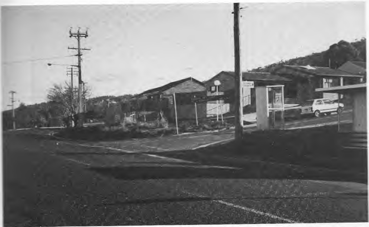
Home Units now occupy the School site. Their foundations were poured in October 1986.
