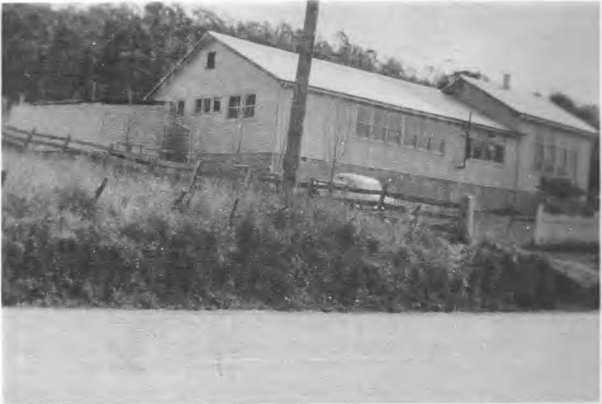
The Coolamon Road State School showing the one-room extension added in 1952 between the 1956-57 extension on the left, and the original building on the right.
