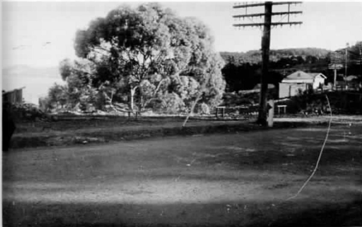
Taken from the bottom of Churchill Road, with the foundations of the old shopping centre being put in and Mr Jenkins' dairy on the site of the hotel. Note: Jenkins Street has not been made, 1949.
