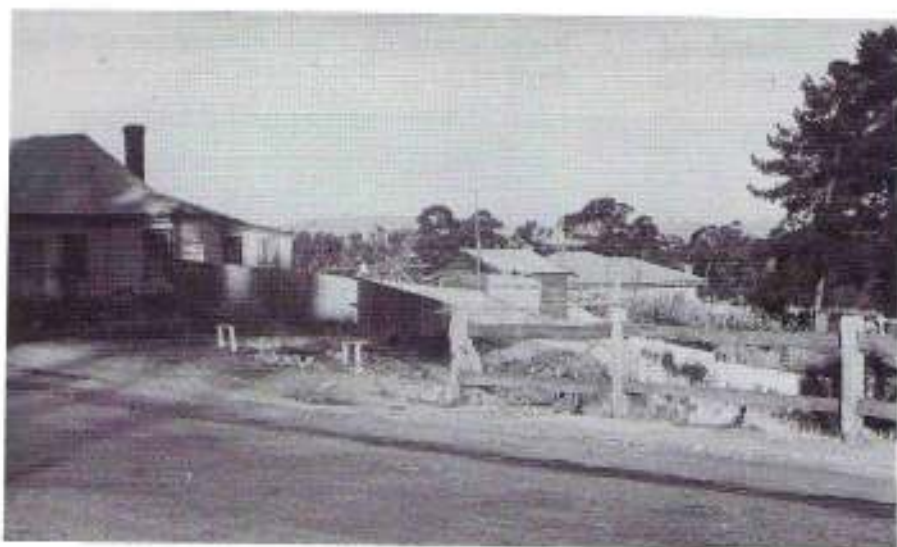
Site of the old shopping centre with the Taroona Tea House on the left, 1949-50
