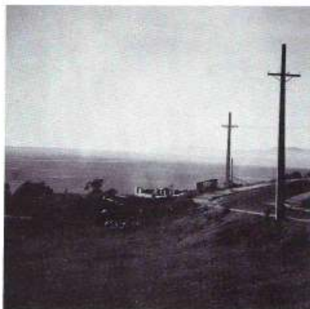
Illawong Crescent looking south, showing the foundations of number 16, the home of Drs Alan and Hilary Wallace.
