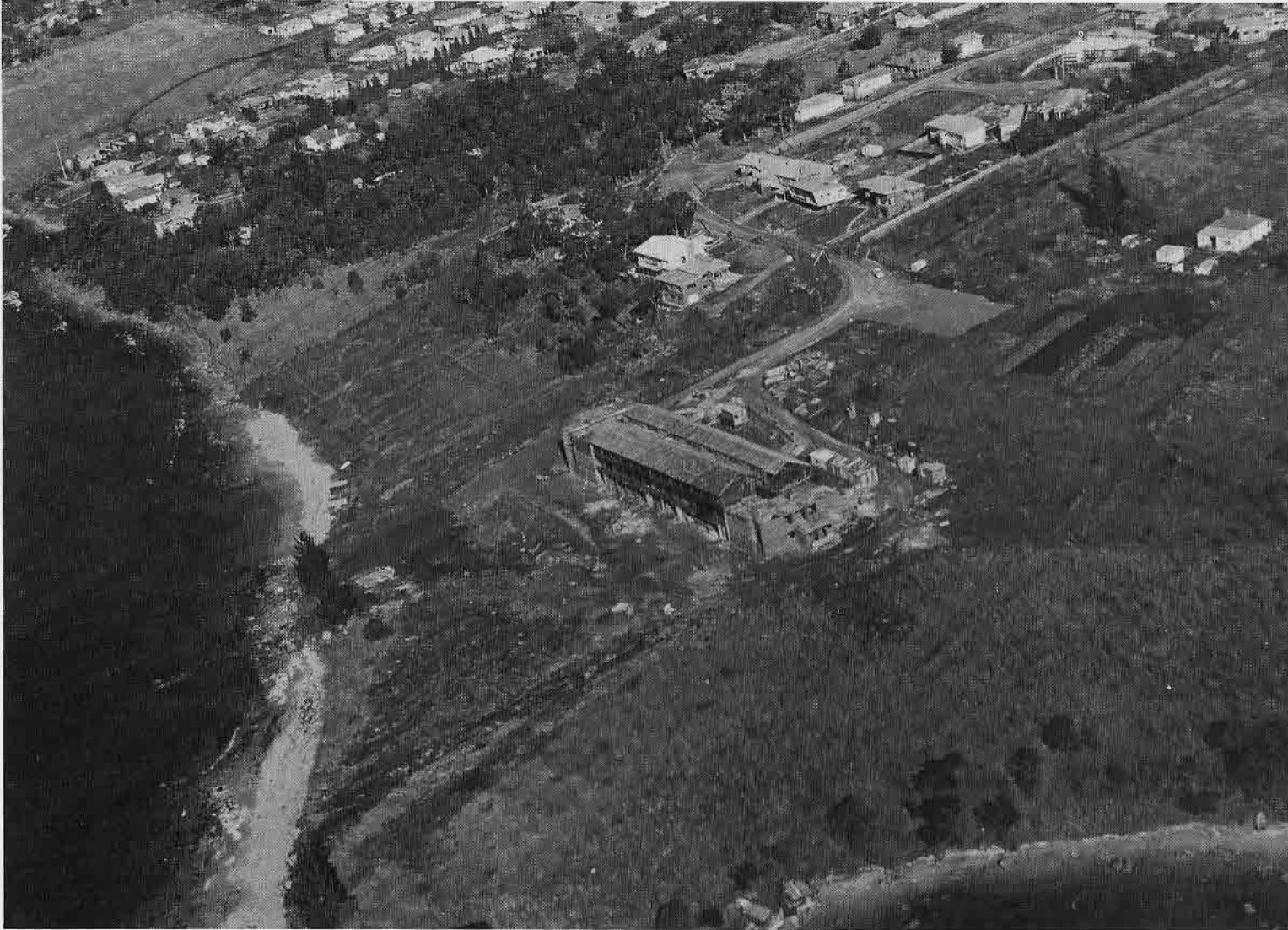
Aerial view of "Retreat Farm" with "A" Block under construction. Mr George Dixon's house in the top righthand corner with Beck's Beach to the left of the pine trees, Dixon's Beach between the pine trees and Retreat Cove in the bottom righthand corner, 1957.
