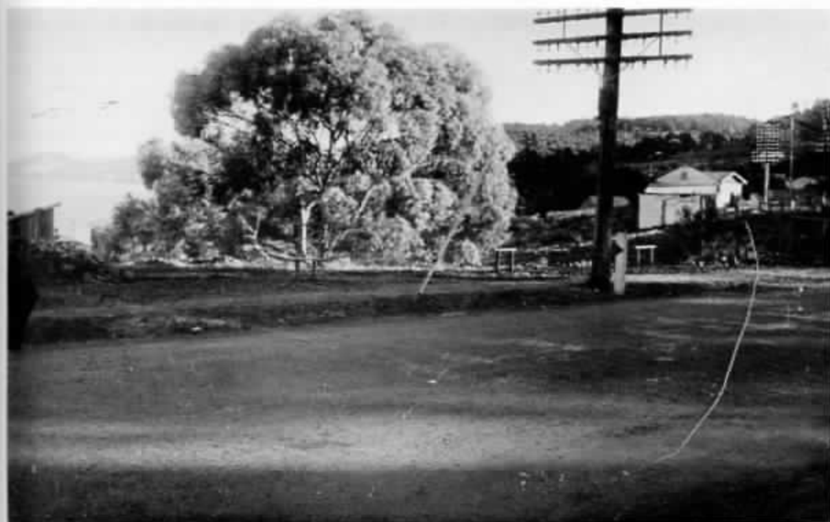
Taken from the bottom of Churchill Road, with the foundations of the old shopping centre being put in and Mr Jenkins' dairy on the site of the hotel. Note: Jenkins Street has not been made, 1949.
